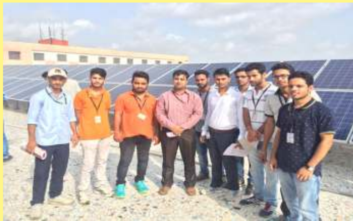
Visit to Roof top Solar Power plant at JIET during Tutor Meeting
